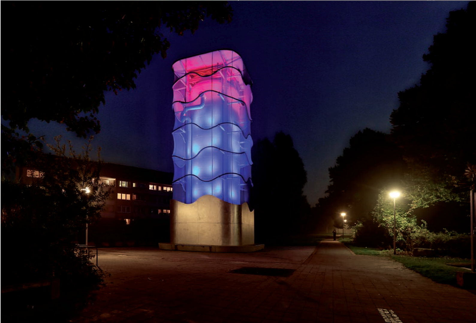
Wärmespeicher (Germany) Photo Credit: SSP Design
